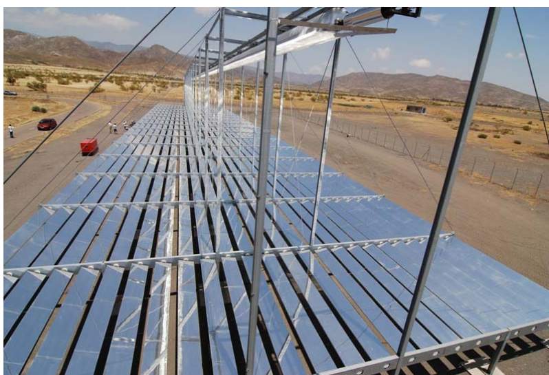
Figure 5.7 Photo of the MAN linear Fresnel demo collector erected on the Plataforma Solar de Almería (PSA).
