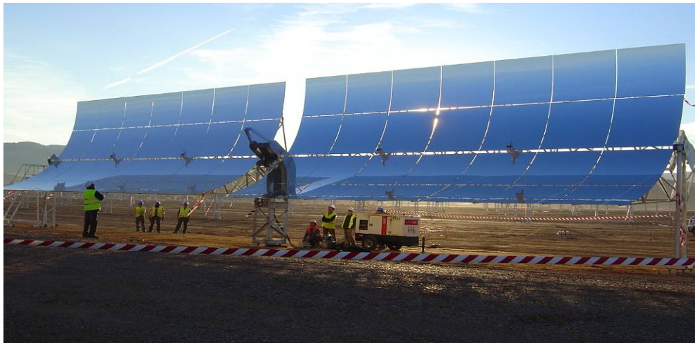
Figure 3.8 Erection of collectors
