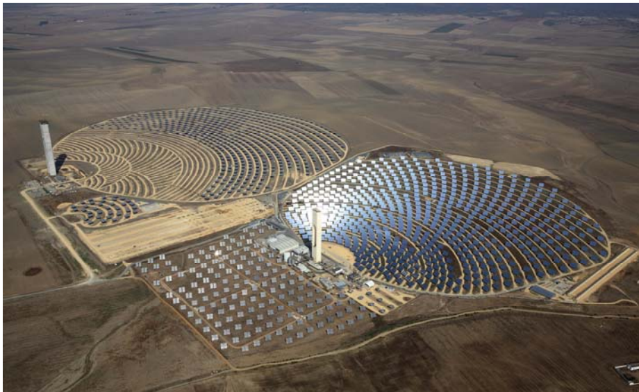
Figure 2.6. View of Abengoa's Plataforma Solar de Sanlúcar la Mayor showing the 11-MW PS10 and the 20-MW PS20 under construction near Seville, Spain
