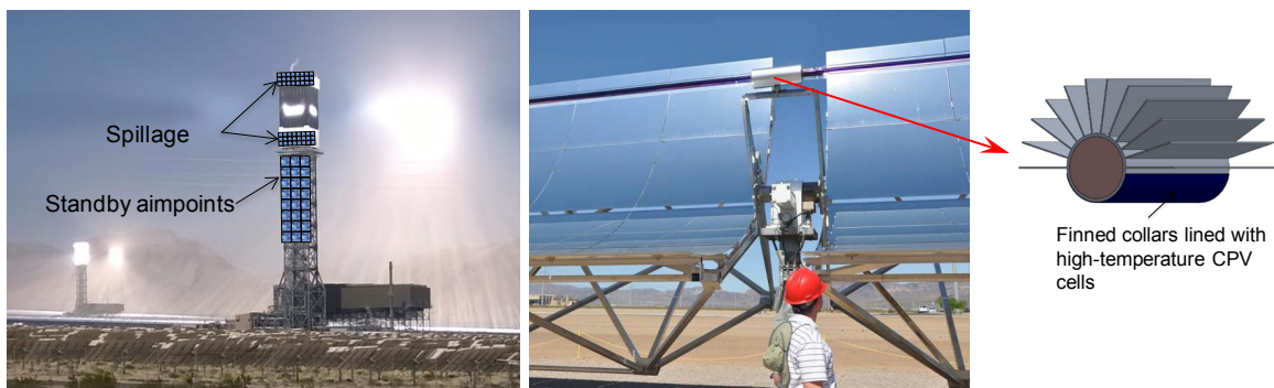
Figure 1. Conceptual design of PV cells on heat shields or standby regions of a central receiver (left) or on the bellows shields of a trough receiver (right).
