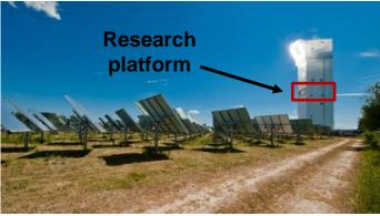
Demonstration on the Solar Tower Jülich ~100 kW total thermal power
