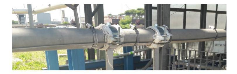
Heating cables fixed by metal clamps
