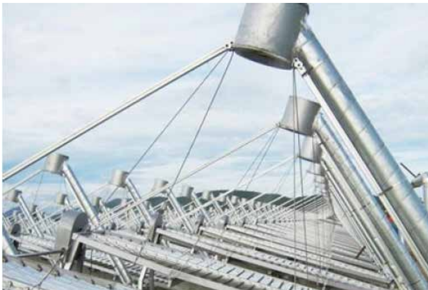
Fig. 4.2-4 Hainan MH-CSP (Source: Network)
