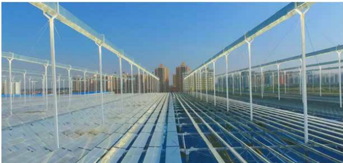
Fig. 4.2-7 1 MW Linear Fresnel Solar Collection System Built on Roofs of the Production Workshops by Lanzhou Dacheng
