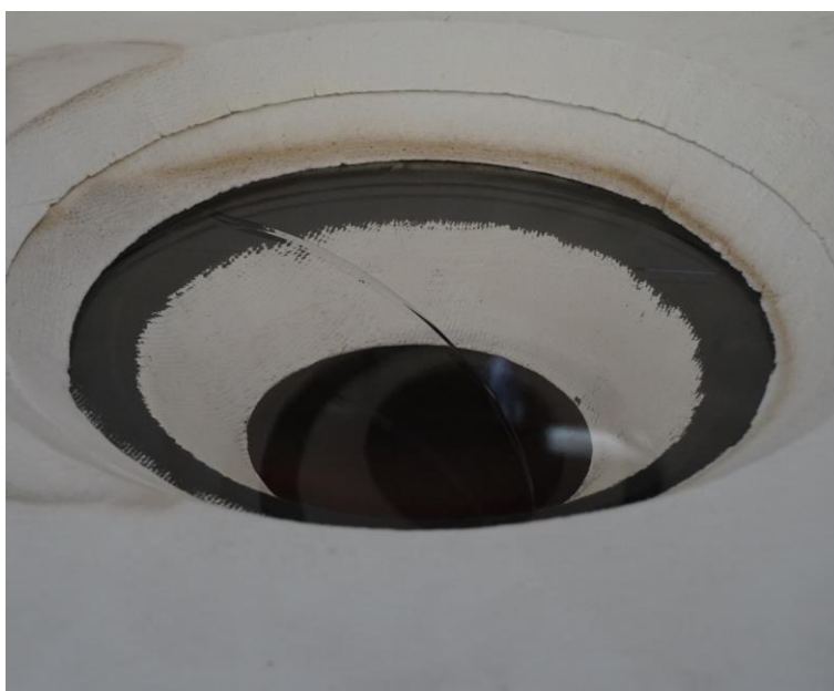
Fig. 125: Crack in the window on February 09, 2017.
