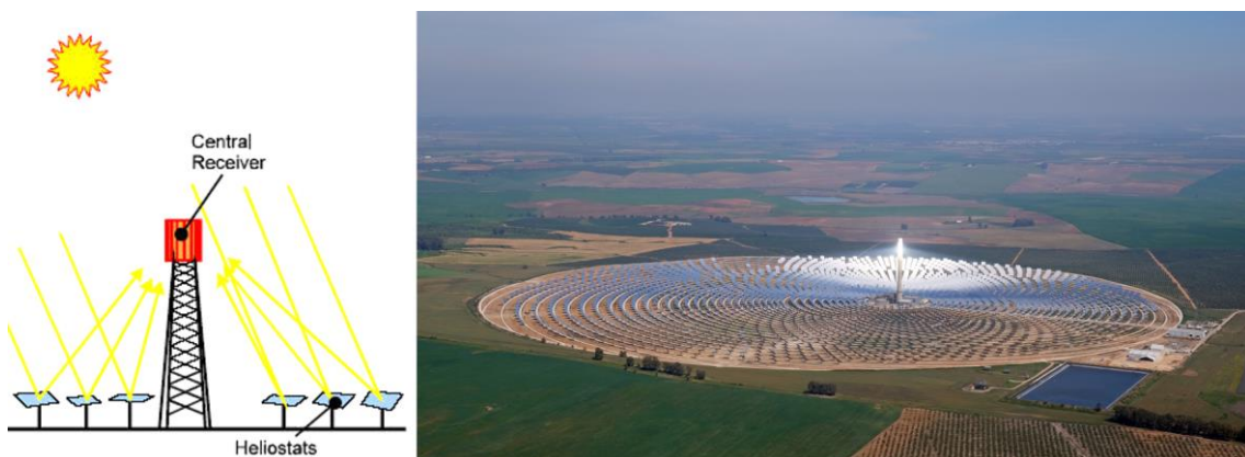
Fig. 22: Solar tower (point concentrating) systems. Left: Operational principle (SolarPACES, 2018). Right: Aerial view of the Gemasolar plant in southern Spain 37 .
