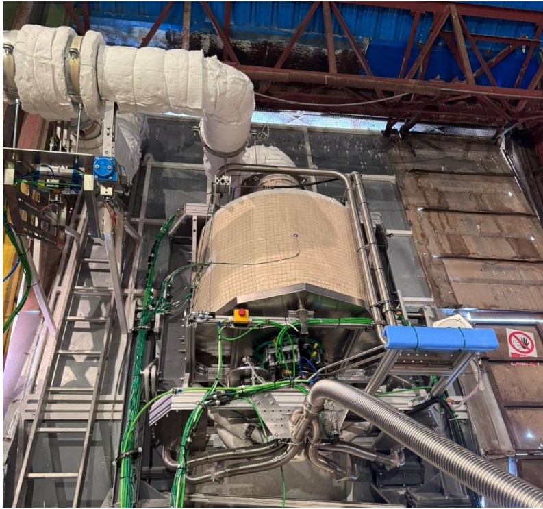
Figure 9: Integrated TRL8 CST system for cost-effective and flexible high temperature industrial heat as demonstrated at PSA.
