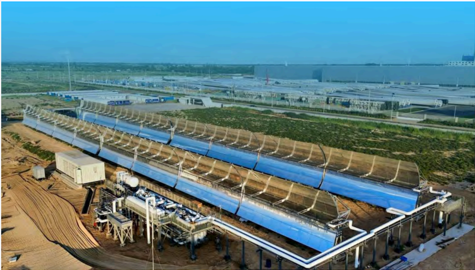
Figure 22: Longteng Solar Molten Salt Trough Concentration and Collection System Verification Platform
