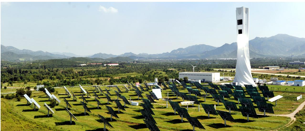
Figure: China's First 1 MW Tower CSP Plant (Source: Institute of Electrical Engineering, Chinese Academy of Sciences, Photographed in 2012)
