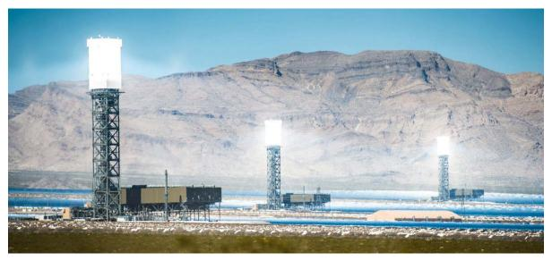
Figure 6-2. Ivanpah water/steam receivers Source: Google Images
