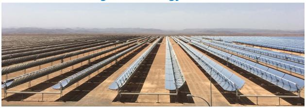
Figure 5-1. 160-MW<sub>e</sub> Noor Ouarzazate I Parabolic Trough Plant, Ouarzazate, Morocco
