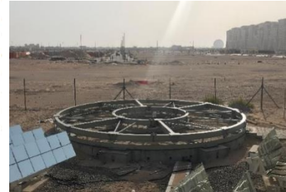
Fig. 5. ASC system turn table operational.
