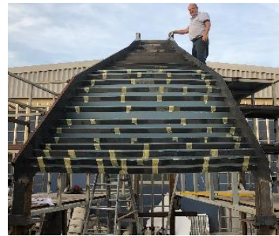
Fig. 3. Construction of 1/16 of the ASC dome.
