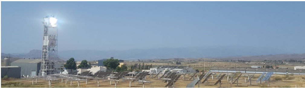
FIGURE 8. SSPS-CRS experimental tower at CIEMAT-PSA during on-sun testing of the CAPTURE prototype
