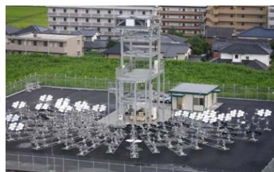
Fig. 2 100-kW th beam-down solar concentrating system at Miyazaki, Japan
