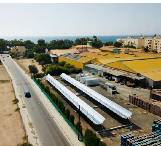
Solar process heat generation at Kean Soft Drinks Ltd. in Limasso, Cyprus. Foto: Protarget AG
