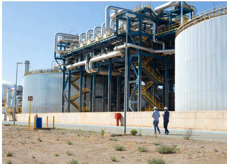
Thermal storage systems decouple the generation of electricity from the 'harvesting' of solar energy. Credit: CSP Services
